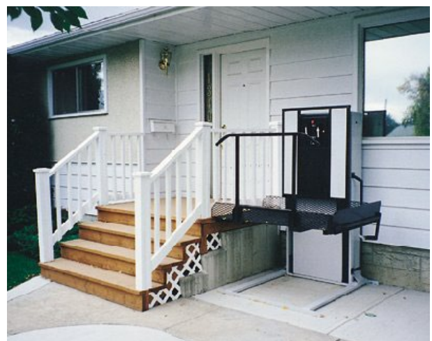
Figure 10. An accessible building entrance that illustrates a functional difference from the stair-based entrance in Figure 9.
