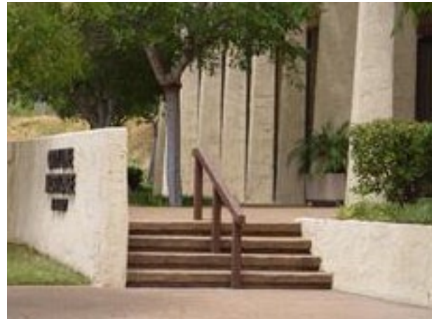
Figure 9. An inaccessible stair step.
