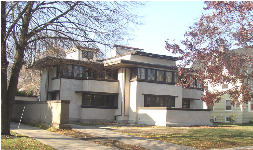
Figure 5. Oscar Balch House, Oak Park, Illinois, 1911, by F. L. Wright. A three part arrangement for the living spaces is reflected in the external organization. Photographer: Damian Trostinetzky.
